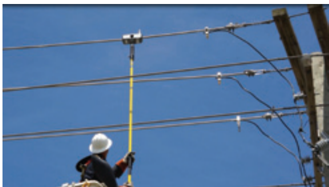
Hot stick installation of smart grid line sensor
