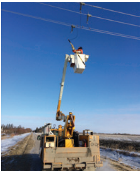
Lighthouse MV Power Sensor installation
