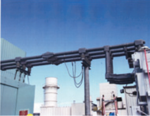
Transformer station with reusable insulating boots encapsulating the 13.8kV transformer bushing terminations, busbar, busbar supports, and expansion joints
